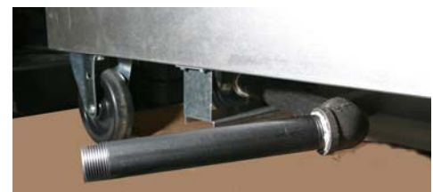
Figure 1: Drain shown extended away from unit cabinet.
